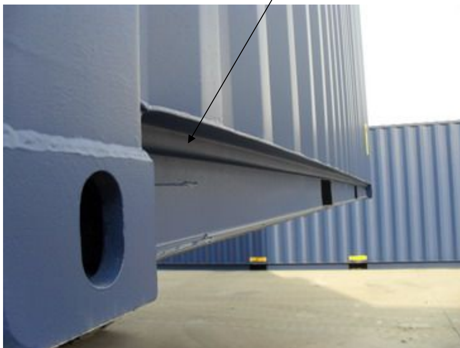
Bottom Side Rail (Double “Z” Section)
